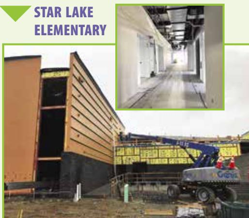
Construction on the new Star Lake Elementary is right on schedule! The drywall installation has been completed in the classroom wing, and the exterior covered play area has been built. Construction crews continue to work on roadway improvements, site grading and more. We're looking forward to scholars occupying the new building in fall 2022.
