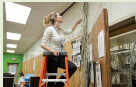
**It's nearly impossible to install wiring for current technology.** The current building can't be easily reconfigured for instructional changes. Here's one example: Throughout Federal Way High School, brick walls restrict wiring for modern technology. Multiple additions have resulted in many interior walls that were once exterior walls. These thick, solid walls add dollar signs to virtually every effort to incorporate modern technology in the school.
